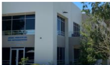
< Van Nuys HQ Facility
